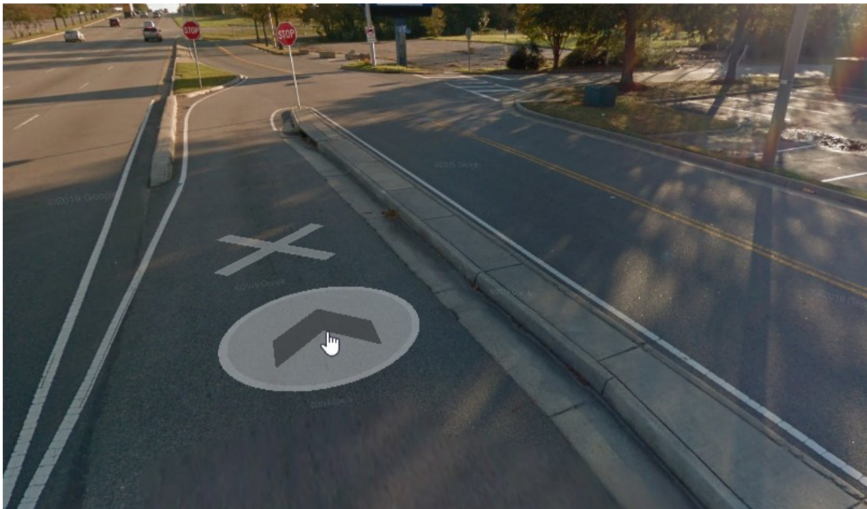
FIGURE 26 - PEBBLE LANE EXIT FROM MILITARY HIGHWAY TO FRONTAGE ROAD
