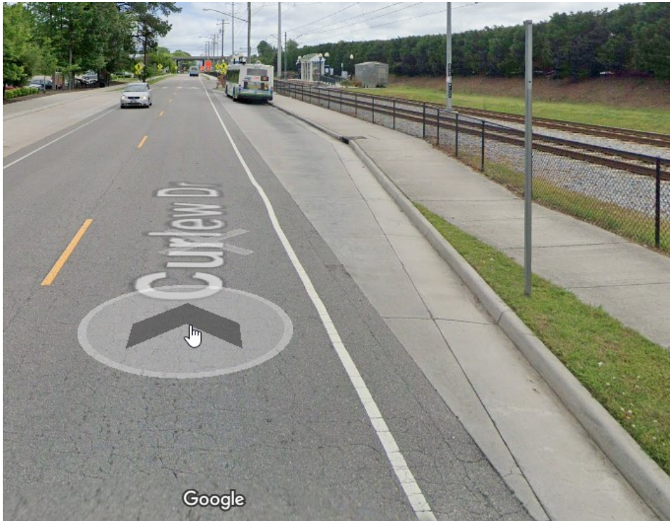
FIGURE 23 – CURLEW DRIVE LOOKING EASTBOUND AT THE PRIMARY BUS PULL-OUT
