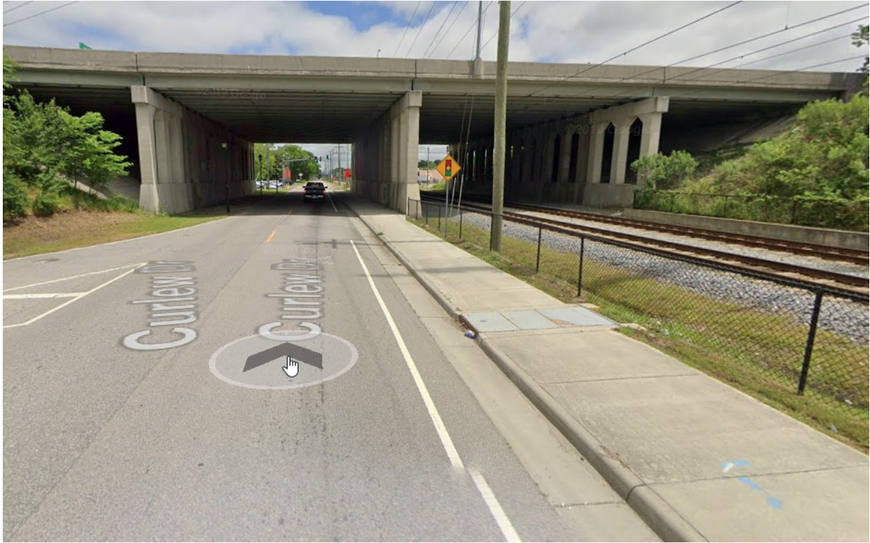
FIGURE 21 - CURLEW DRIVE AT MILITARY HIGHWAY FRONTAGE, LOOKING EAST
